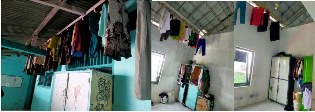
Fig 1. Condition of Dormitory Room Before Intervention Source: Personal documentation (2024)
