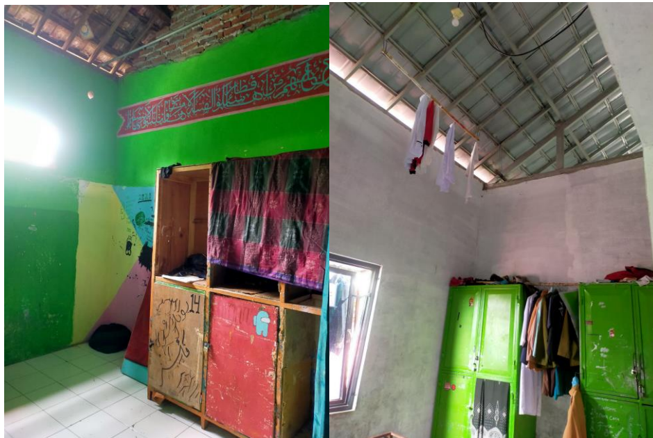
Fig 2. Condition of Dormitory Room After Intervention (same room) Source: Personal documentation (2024)
