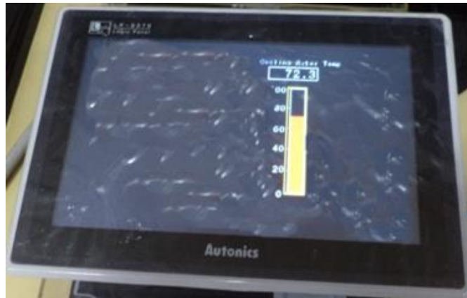
Figure 10. Main Engine Cooling Water Test
